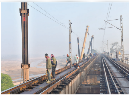
24 X 12.2m + 4 X 27m Span at Madankatta, Jharkhand
