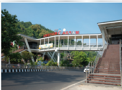
Foot-Over Bridge at Kamakhya Gate, Assam
