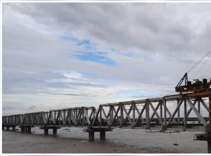
15 X 61m OWG Cantilever type erection at Kursela, Bihar
