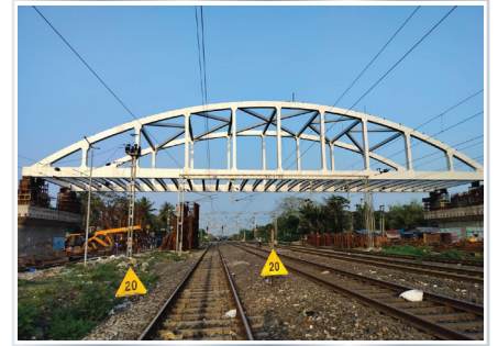
1 X 60m Span Bow String at Basugaon, Assam
